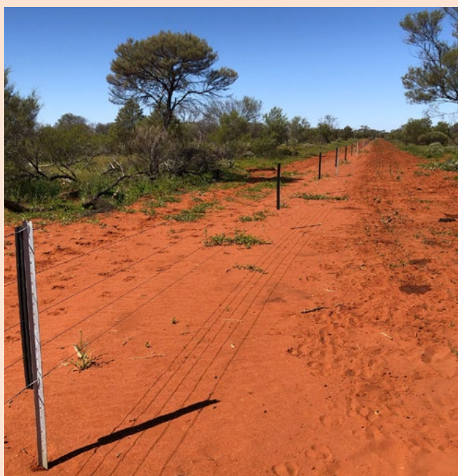
Image 3 Westonfence 5-wire electric fencing (pictured here) and 8-strand electric fencing was used to fence off the 9,000 ha demonstration paddock
