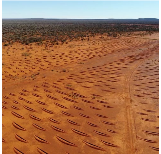
Image 10 Image of the hard pan seen in Image 9 after installing grader scallops
