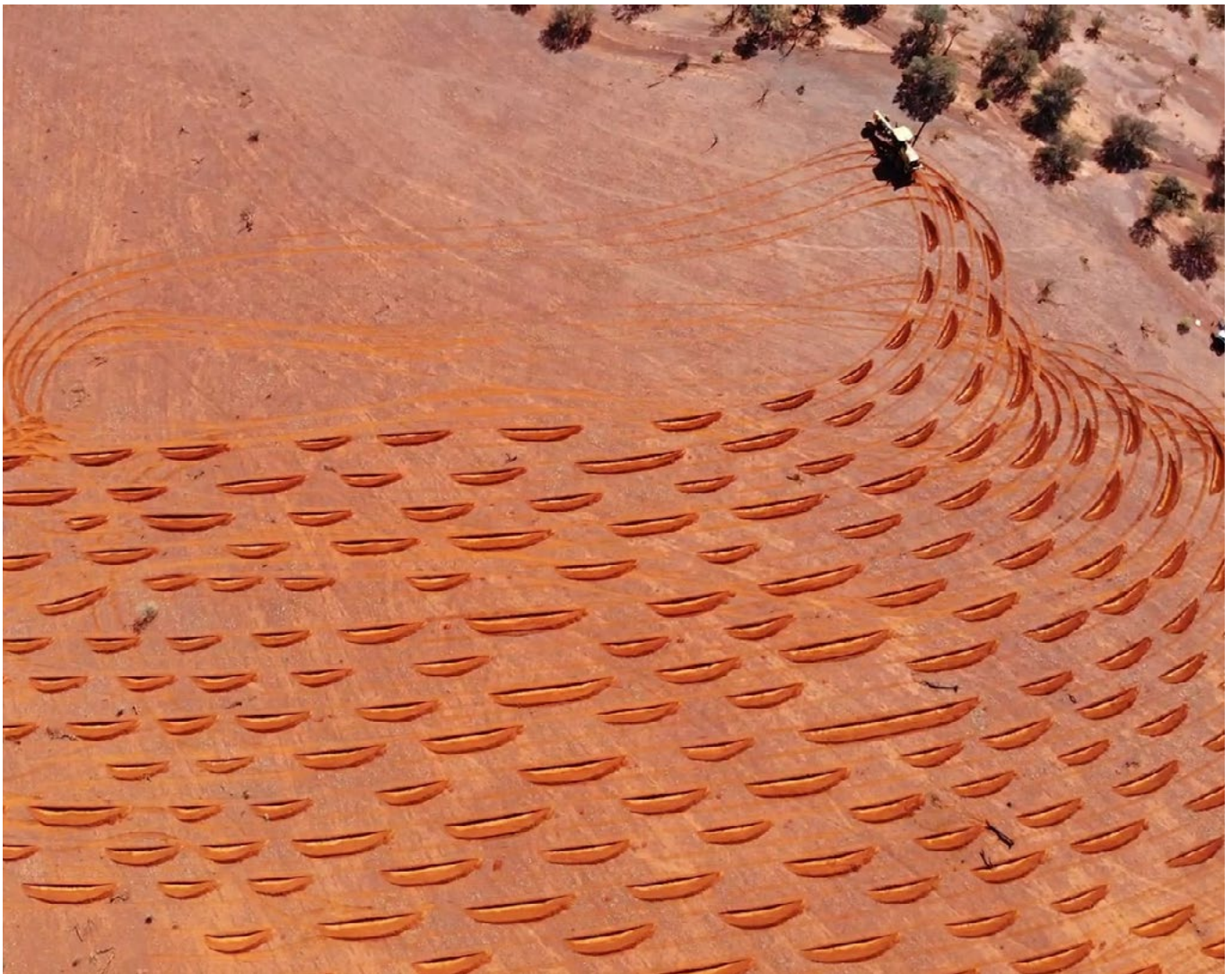
Image 11 Creating grader scallops on Challa Station to slow and trap water, soil and seeds
