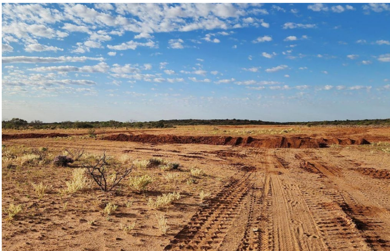
Image 13 Installation of low track bunds on the new track
