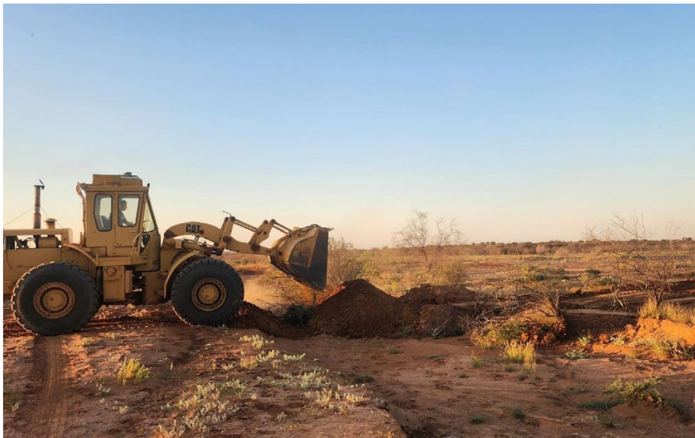
Image 10 Remediation of unused section of track with scrub sieves. James Baston using the loader to provide cover to scrub that has been packed
