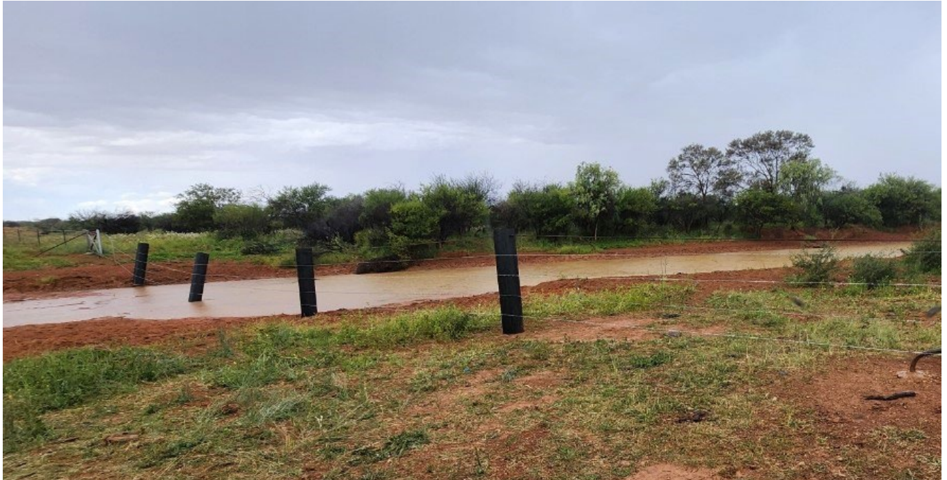
Image 2 'Floating fence' built across the Jacobs Gully creek line
