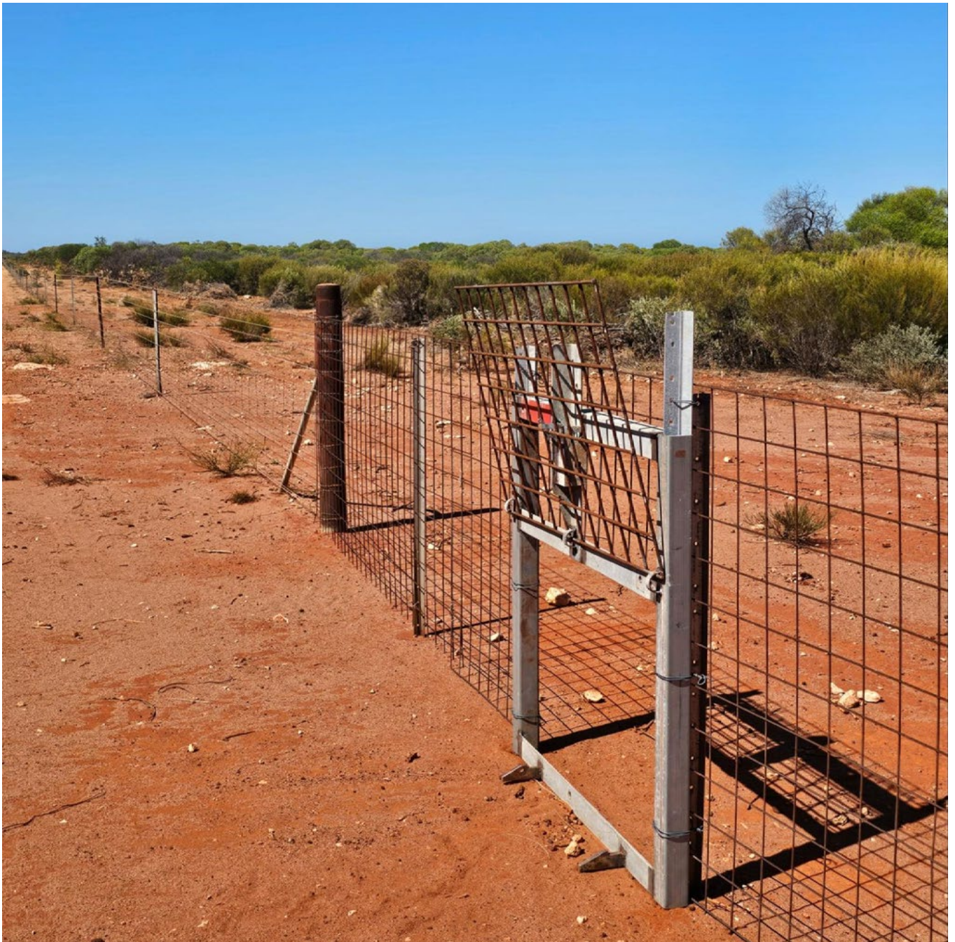
Image 2 Calum designed these ‘goat gates’ which he installed in the fence to allow goats through and prevent damage to fences Source: Belinda Carruth
