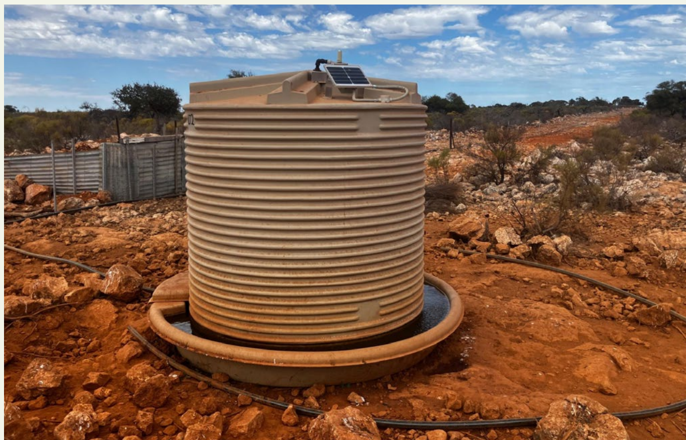
Image 12 Remote water flow-in and flow-out meters are installed on the tanks and troughs in the linear trap yard Source: WA DPIRD
