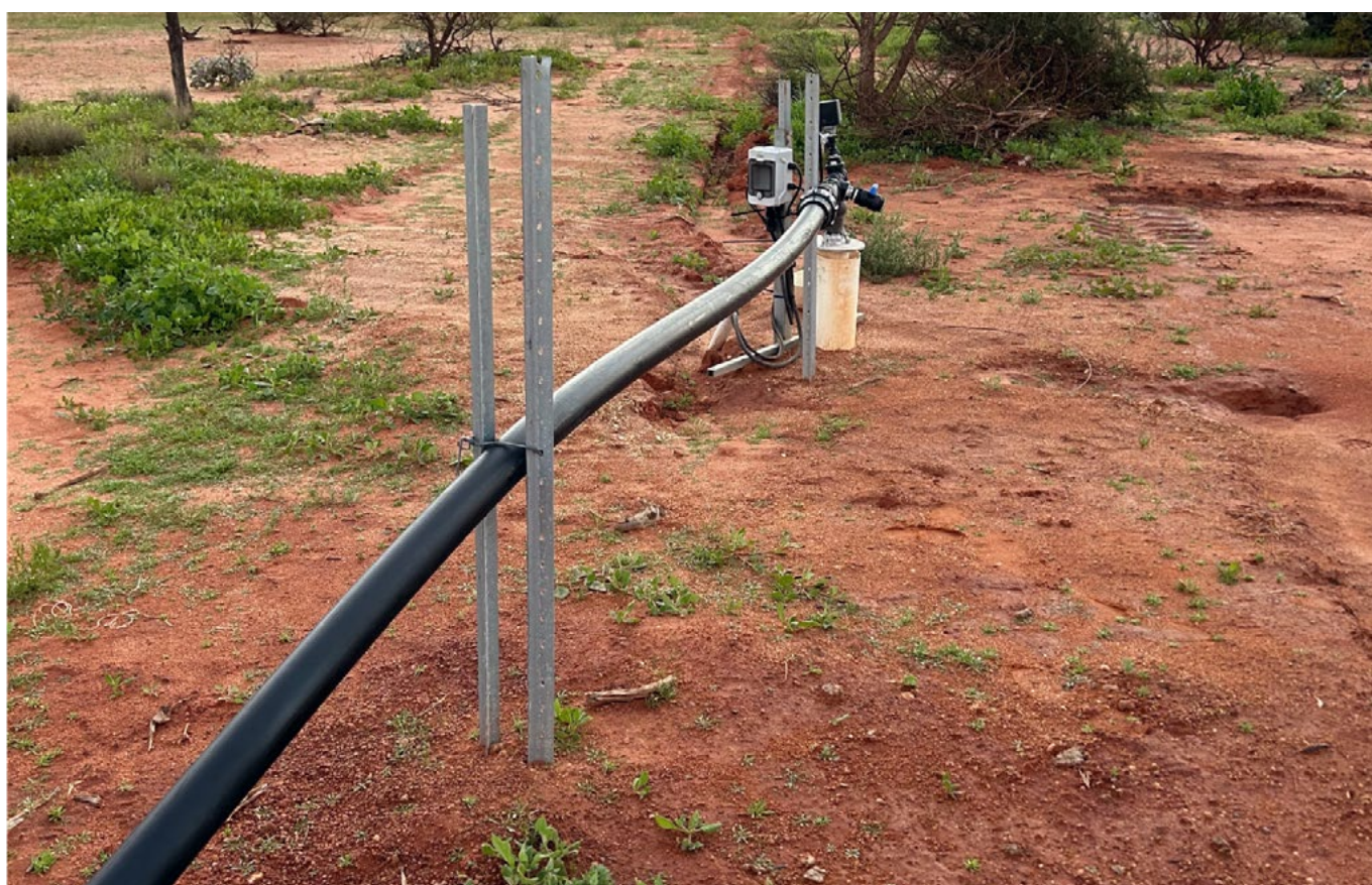
Image 4 The new bore drilled to 37 m that supplies water to the 200,000 L tank at the top of the hill Source: WA DPIRD
