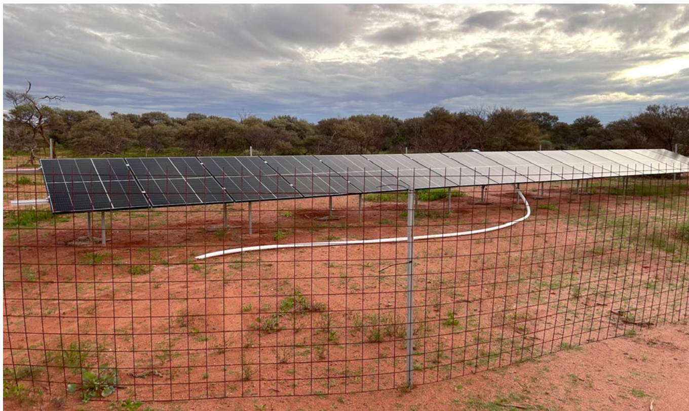
Image 3 7 kW solar system to power the new bore, which pumps water 6.5 km up to a 200,000 L holding tank Source: WA DPIRD
