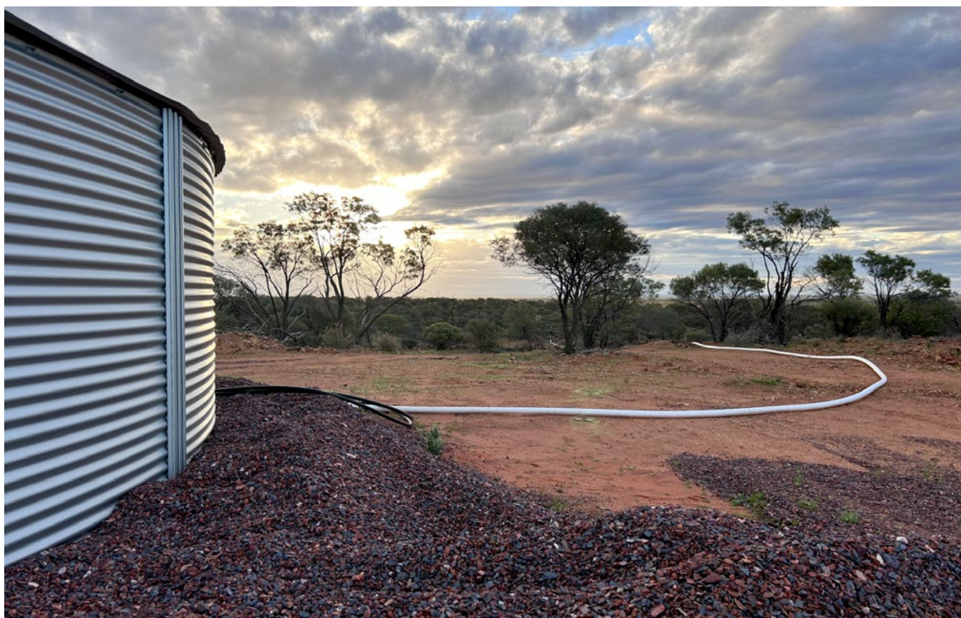
Image 5 Water stored in a 200,000 L tank at the top of a catchment funnels down 17 km of poly pipe to a series of 12 tyre troughs Source: WA DPIRD
