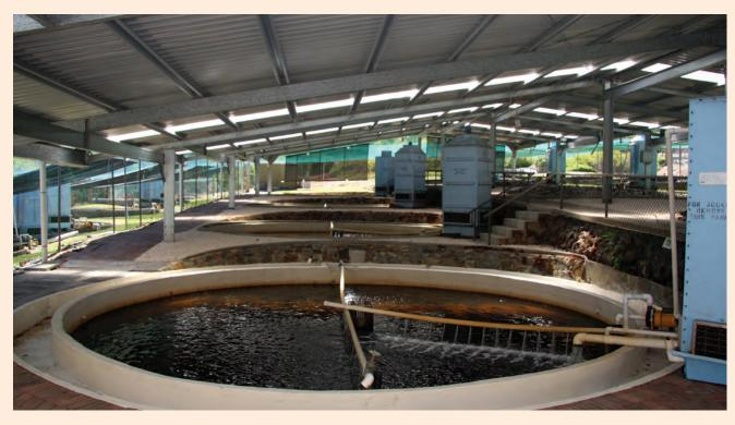
Hatchery ponds were covered with a roof in 2003 and evaporative cooling towers (blue boxes) installed to reduce water temperature during summer.
